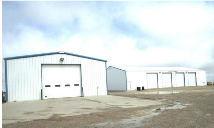
NodalSeismic's new headquarters located in Dighton, Kansas.
